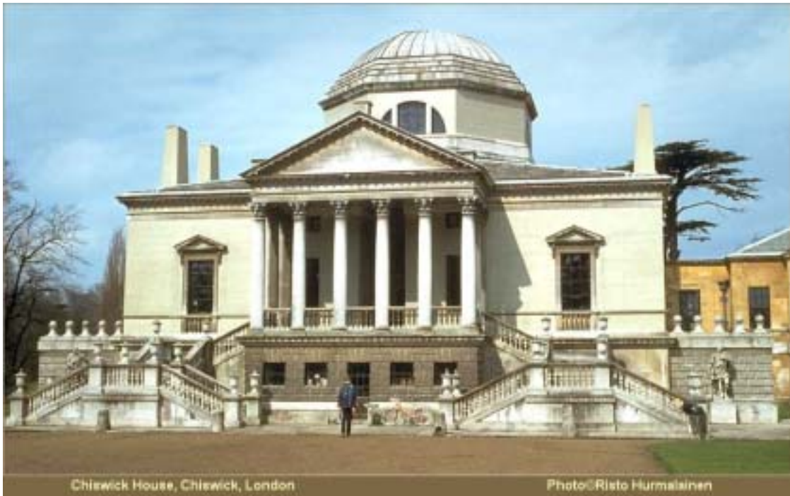
Lord Burlington and William Kent, Chiswick House , 1729 (stone) (Chiswick, London)
